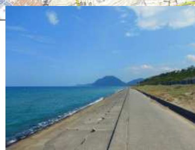
踏査地点03-6 (土砂投入場所東側)
